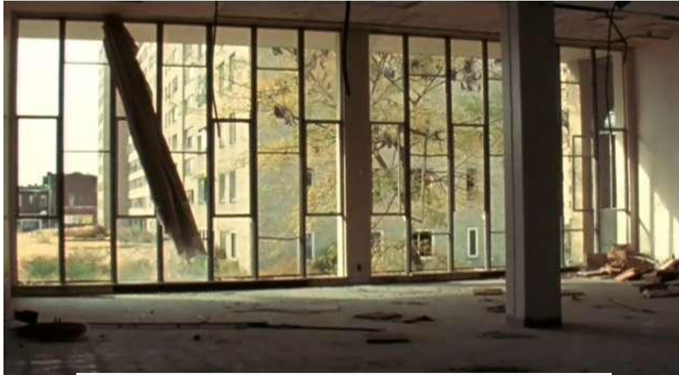
(From inside one of the notorious common area breezeways)
